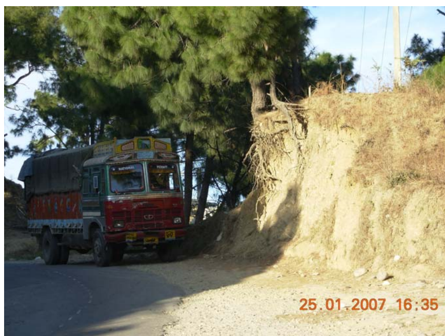
Exhibit 11 Road side trees posing a hazard to road users along Una-Barsar-Jahu -Nerchowk
