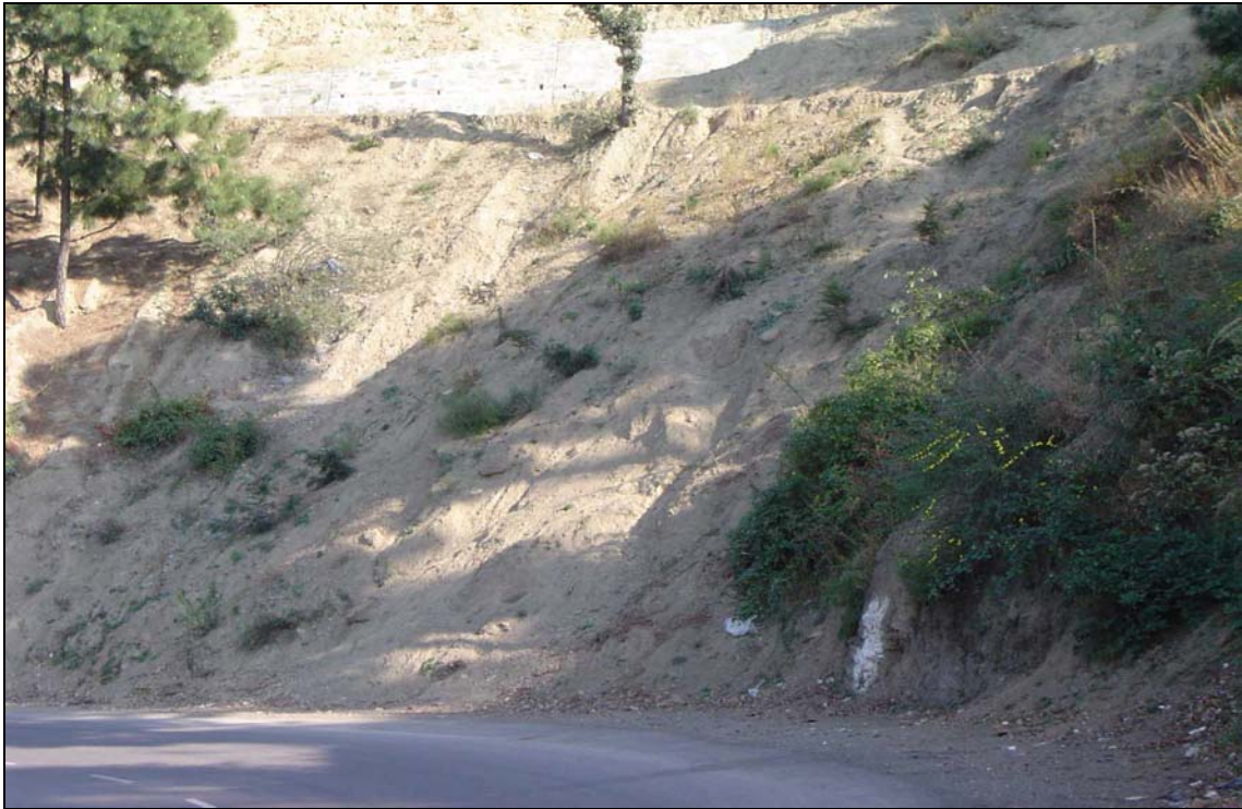
Plate 2. A typical roadside slope failure, caused by careless spoil disposal.
