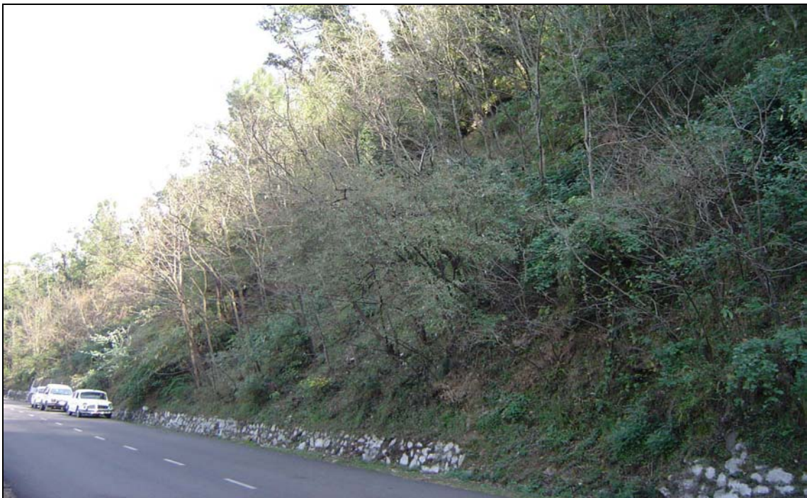
Plate 5. A Slope Stabilised by Planting Undertaken by the PWD's Horticulture Wing under a previous initiative.
