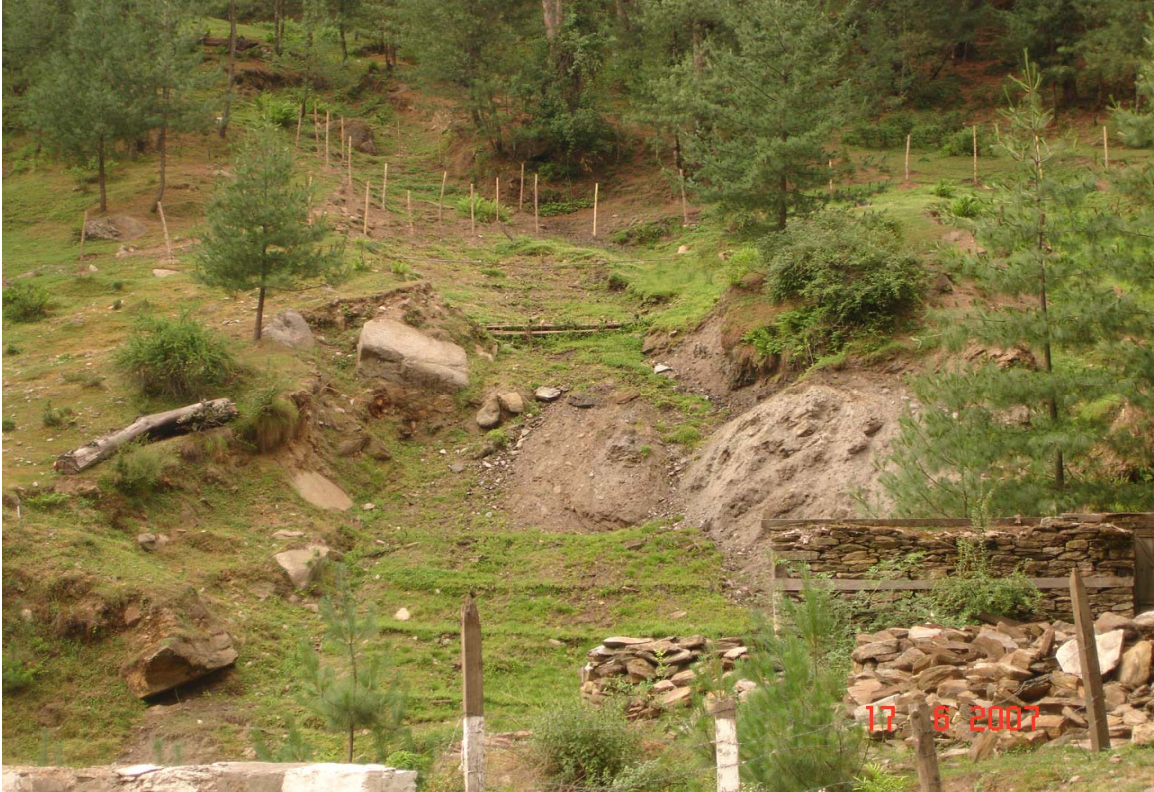
Plate No. 1: Close view of the Sundali nala gully and performance of the plant growth after 6 months of bioengineering construction
