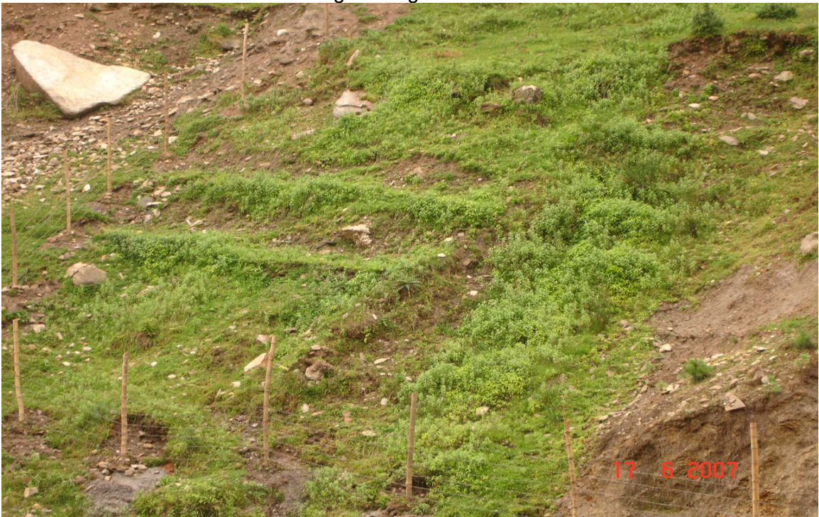
Plate No. 2: Close view of the brush layering technique behind the barbed fence in Sundali nala gully and performance of the growth after 6 months of bioengineering construction.
